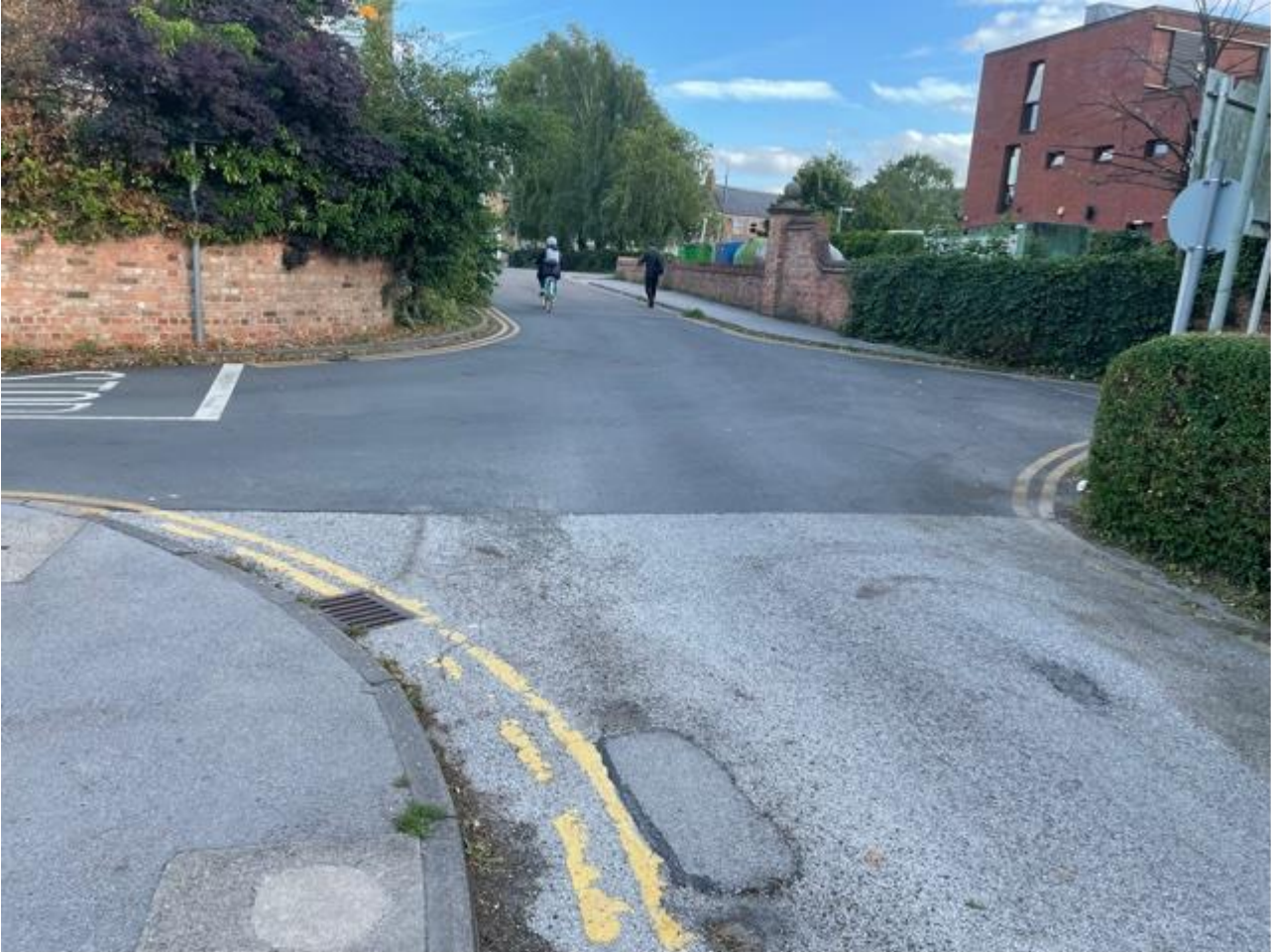
Picture: The Accessway
